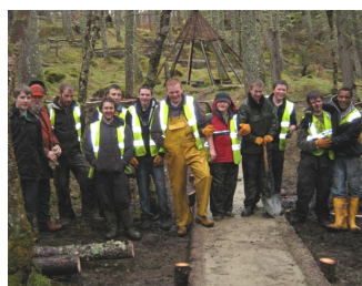
The finished section of path
