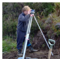
Setting out the foundations for the shelter
