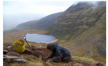
Filling in the gullied section up to Sail Gharbh. Photo: Sandy Maxwell (JMT)
